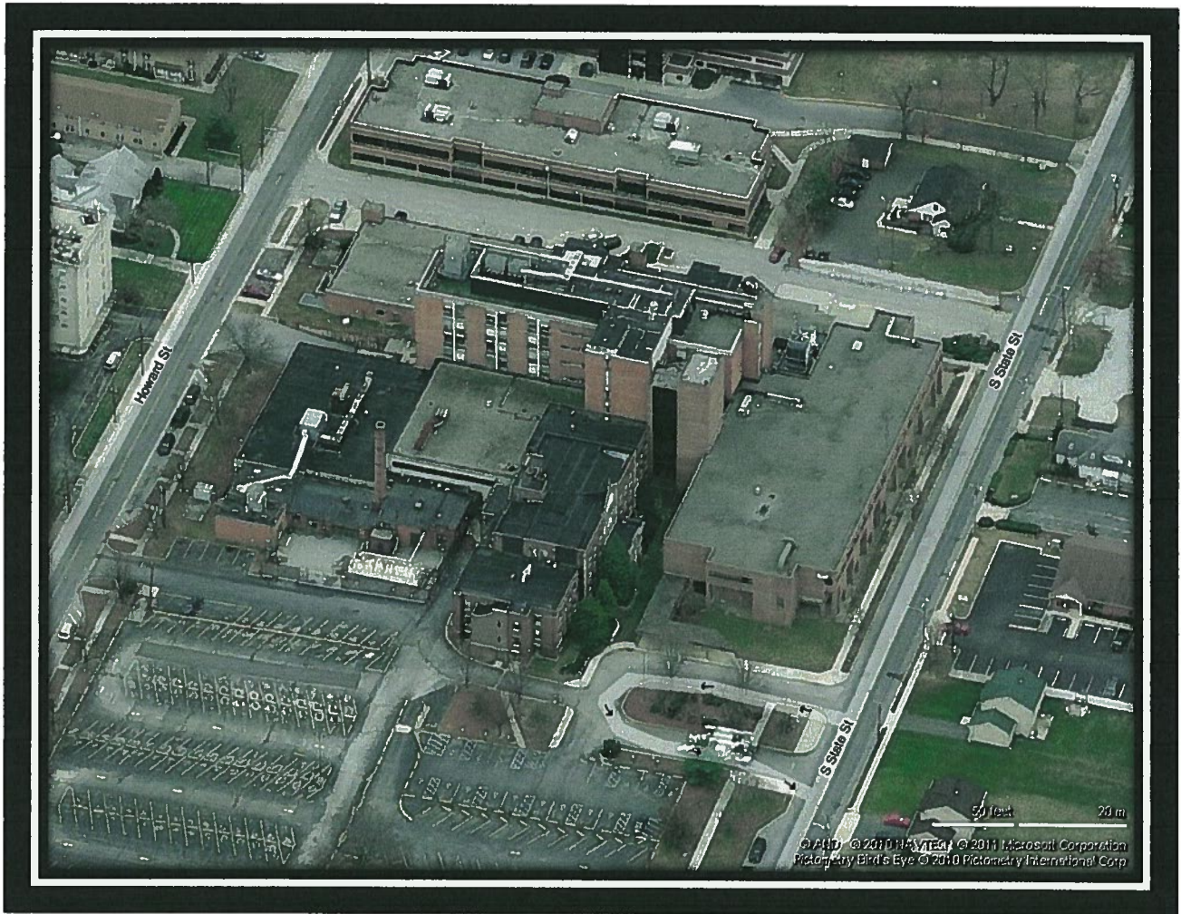
Figure 4 – Newcomb Hospital North Facade
