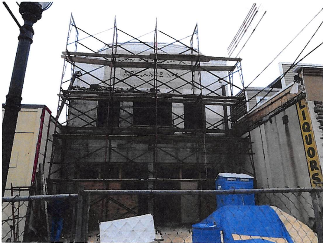
Photograph 1: East elevation of Elks Lodge
