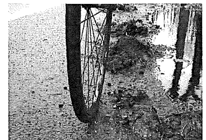
Debris on the Road
