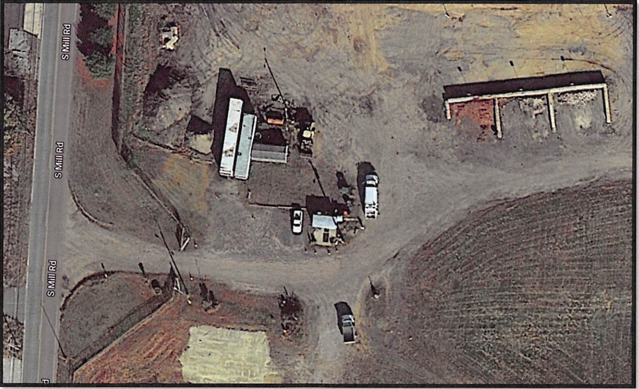
FIGURE 5 Municipal Landfill – Mill Road utility area
