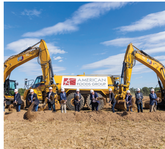
American Foods Group breaks ground in September 2022 on its new facility in Missouri. The company plans to be fully operational by the end of 2024.
